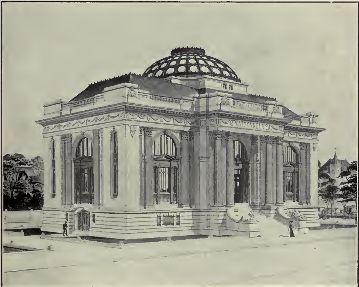
THE POST OFFICE UNDER CONSTRUCTION AT MAISONNEUVE.
